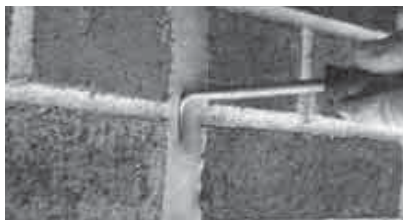
FIGURE 3.9 – SEALANT ADHESION PROBE TEST
