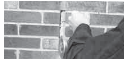
FIGURE 6.1 – USING A PORTABLE GRINDER
