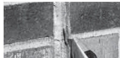
FIGURE 6.2 - USING A RAZOR KNIFE
