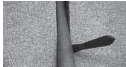
FIGURE 7.1 – INSERTING BACKER ROD
