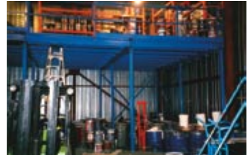
Mezzanine Installation Over Pallet Racking
