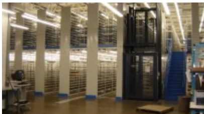
Shelving Supported Catwalk
