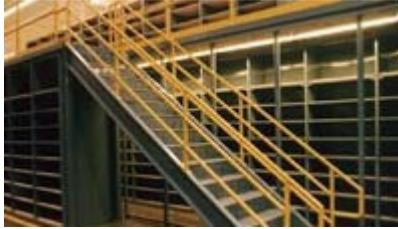
Shelving Supported Catwalk
